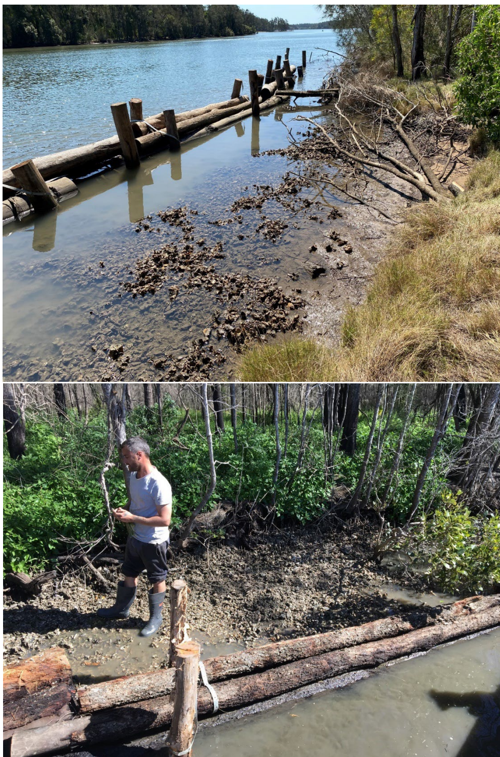
Figure 43. Several projects on the mid north coast completed by the Hunter Local Land Services use oyster shell in combination with timber as a softer erosion control option working with nature (B. Hughes Hunter LLS)
