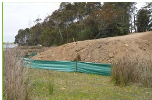
Sediment curtain in place to help stop soil from washing into nearby creeks source: OceanWatch Australia
