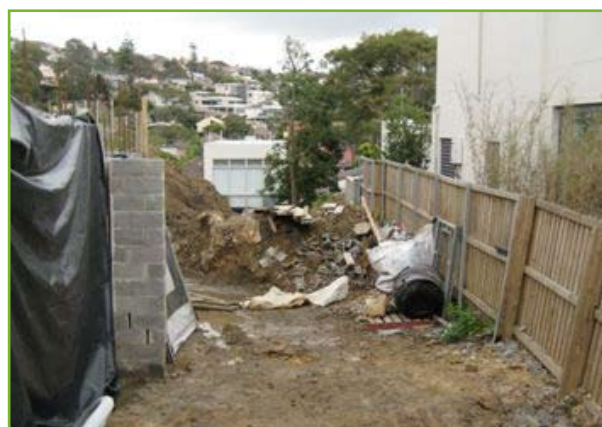
Soil erosion on building and infrastructure sites can be a major source of sediment pollution in waterways. A single building block can lose four truckloads of soil in one storm event, source: OceanWatch Australia
