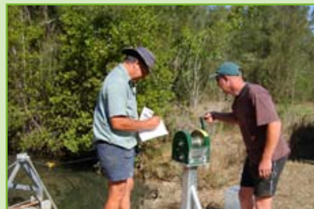
Landholders opening a winch to improve flushing of the drain and thus improve water quality, source: Clarence Valley Council
