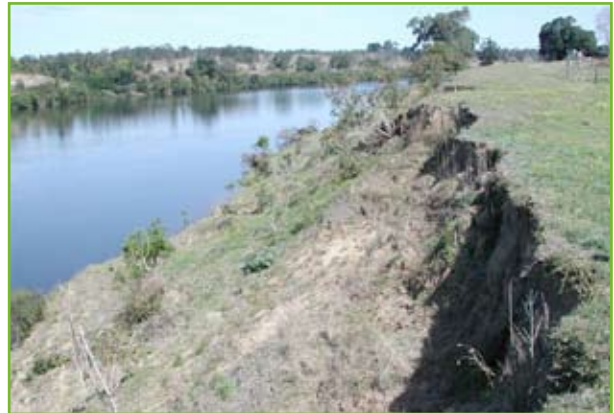
Cleared riverbanks showing signs of erosion, Clarence River NSW, courtesy of DECC
