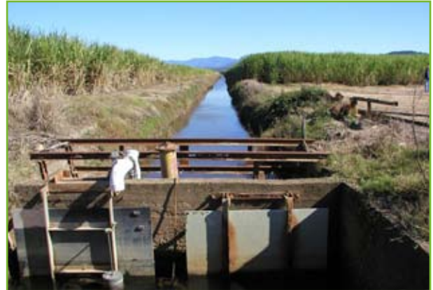
Floodgates closed to stop floodwaters flowing onto sugar cane fields on the floodplain, source: OceanWatch Australia
