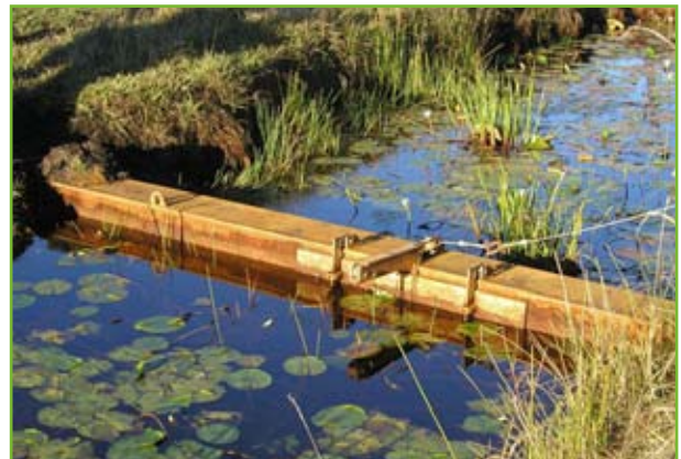
Weir across a creek, source: OceanWatch Australia
