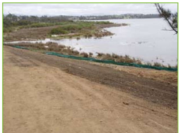
Removal of vegetation cover exposing soil to erosion, South Coast NSW, source: OceanWatch Australia
