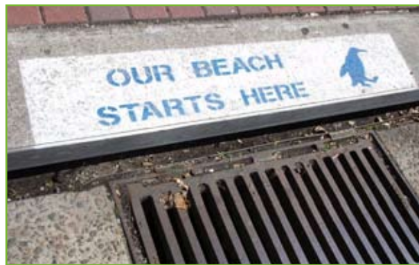
Roadside gutters and drains collect stormwater which then flows through pipes that discharge into creeks, rivers, the ocean or other waterways, source: OceanWatch Australia
