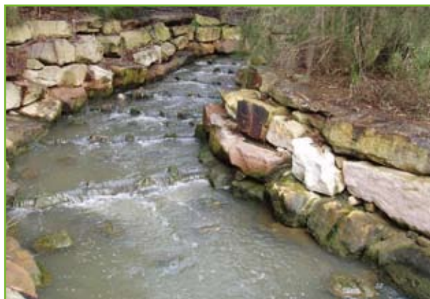
Fishway built such that fish can move around structures such as weirs, Lane Cove National Park NSW, source: OceanWatch Australia
