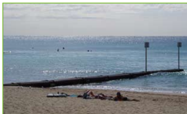
Pipe carrying stormwater from gutters and drains and emptying in the ocean, Manly NSW, source: OceanWatch Australia
