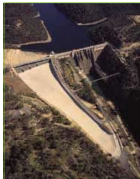
Warragamba dam, source: Sydney Catchment Authority
