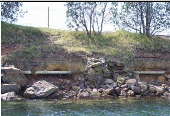
A Destruction of rock retention wall in the southern part of the road bridge that crosses Merimbula Lake at the entrance of the lake
