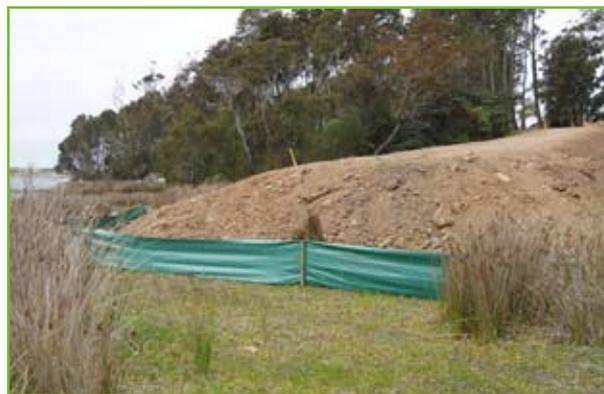
*Sediment curtain in place to help stop soil from washing into nearby creeks source: OceanWatch Australia*
