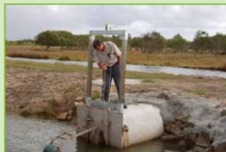
A tidal floodgate with a winch which allows for improved water exchange, source: Clarence Valley Council
