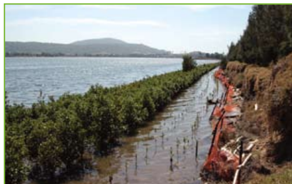
Planting mangroves to help stabilise eroding banks of the Shoalhaven River, source: SRCMA, (Peter Pigott)
