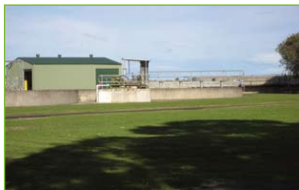
Nowra Wastewater Treatment Plant, source: OceanWatch Australia
