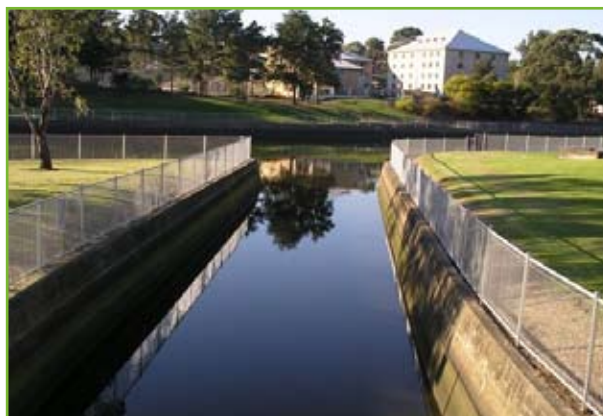
Concrete lined channel, Cooks River NSW, source: NSW DPI (Scott Nicholls)
