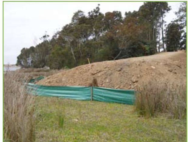
Sediment erosion controls, South Coast NSW, source: OceanWatch Australia
