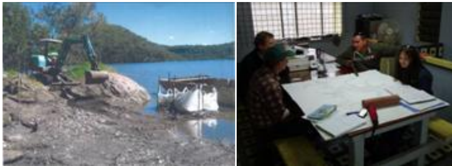
Left: Using a barge and excavator to bag up asbestos.
