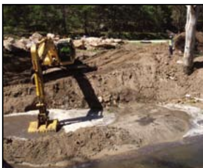
Bank stabilisation and fencing for horse exclusion on Popran Creek
