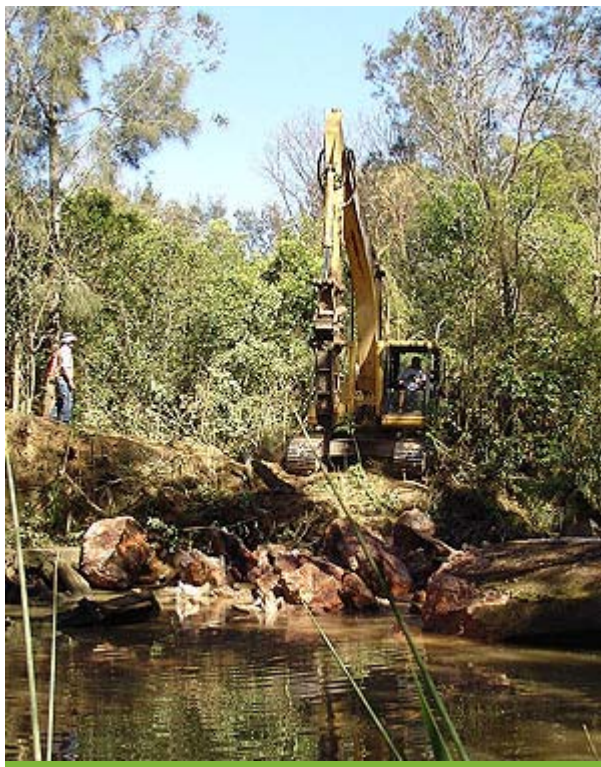
Photo: The redundant weir being removed and opening up fish passage.
