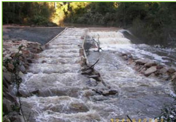
Rock ramp fishway, Karuah River NSW, source: NSW DPI (Scott Nichols)
